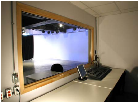
Control room looking into studio 1 < C >
